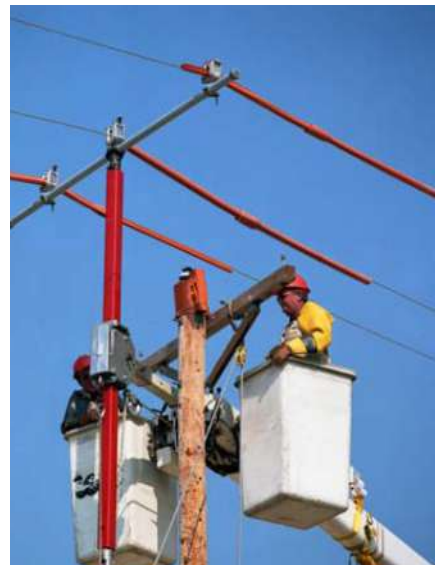
Sleeve for square jib fits other brands of material handler vehicles. Notice, too, that center wireholder may be used alone for single-phase lifts.
