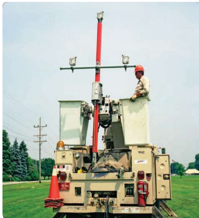
For armless construction, shorter crossarm mounts midway with single wireholder at top of mast. Notice, too, that center wireholder may be used alone for single-phase lifts.
